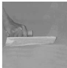
Float the grout material
